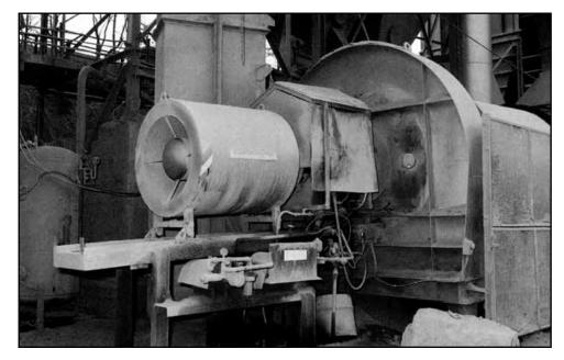
Figure 8 Use of silencer on burner
