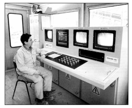
Figure 7 Use of CCTV in a control room
