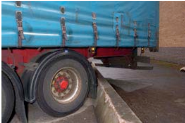
Figure 7 Concrete wheel stop
