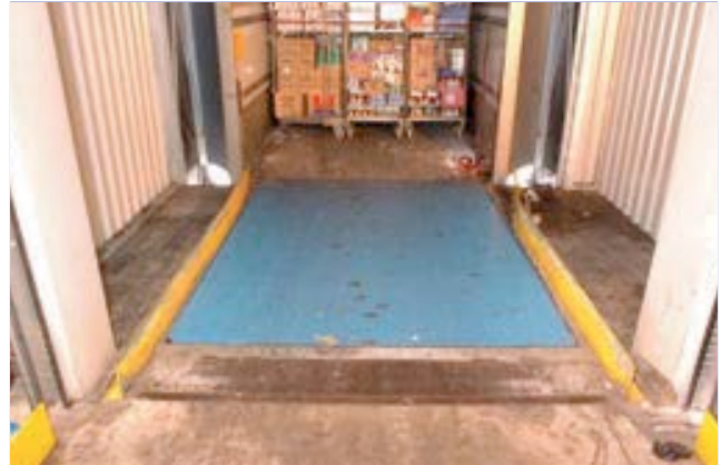
Figure 14 Dock leveller
