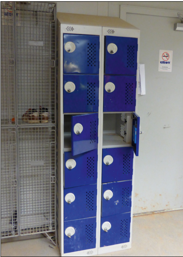
Figure 3 A secure, lockable battery charging point
