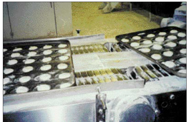
Problem: original metal track conveyor
