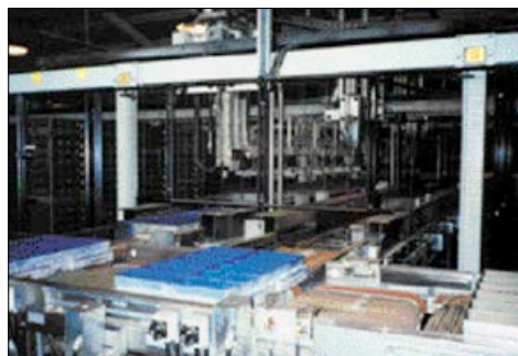
Solution: new robot installed to change tins
