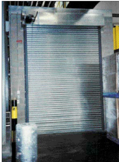
Solution: entrance to the new segregated enclosure for cap storage and delivery
