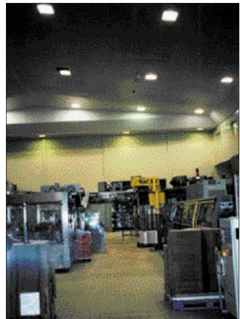
Solution: new design of building with high ceiling and acoustic wall panels
