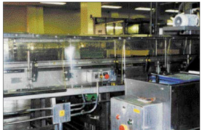
Solution: conveyor with enclosure fitted
