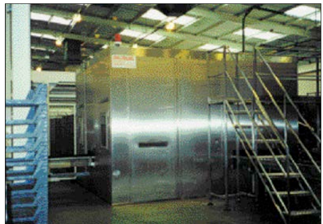
Solution: soundproof enclosure erected around noisy plant
