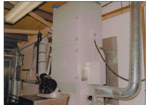
**Figure 18** Dust extraction at flour sack-tip point
