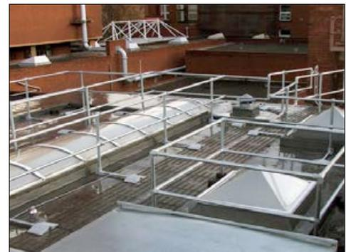
Figure 7 Skylight and roof edge protection
