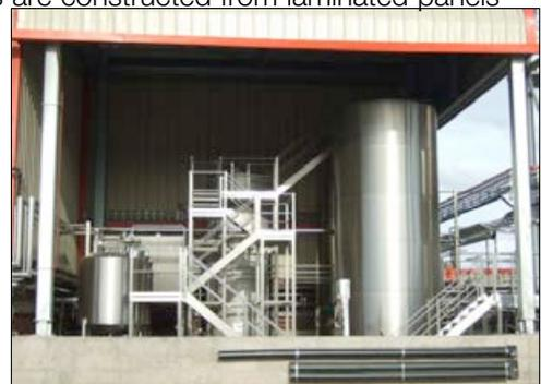
Figure 4 Fixed access system integral to new plant
