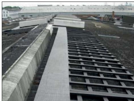
Figure 6 Walkway and fallboards on fragile roof
