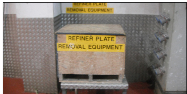
Figure 25 A storage box for tools and equipment
